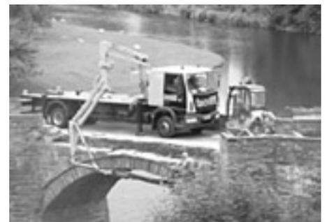
Work on Pont Carrog proceeding with the aid of the 'cherry picker'. The picture also reveals the original bed of the roadway and the immense thickness of tarmacadam which has built up over the years.
